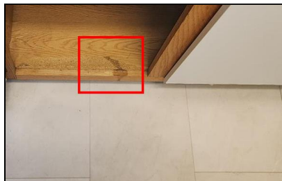
1.0 Item 6(Picture) Example/ Sample- Kitchen Sink
