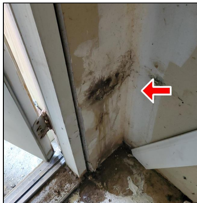
1.0 Item 4(Picture) Example/ Sample- shed
