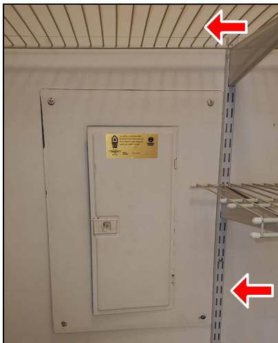
3.3 Item 2(Picture) – consider removing some of the wire rack system considered a typical finding and rarely corrected
