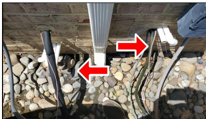
4.5 Item 1(Picture) Located at the front of the condominium building
