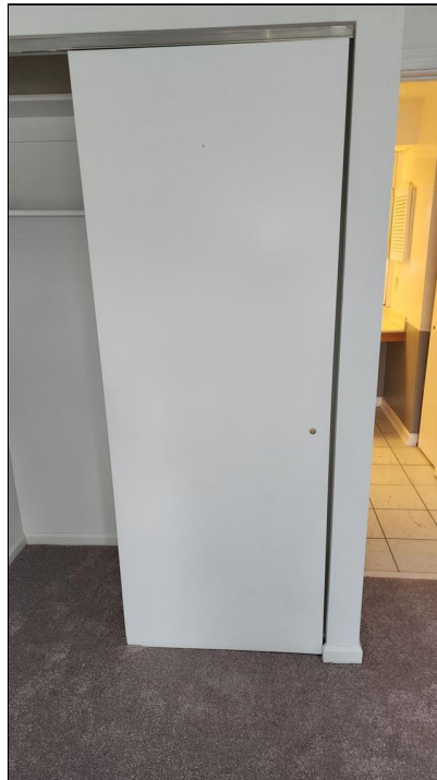
1.2 Item 2(Picture) Example/ Sample- Primary Bedroom Closet- Closet door does not open properly, rubs floor, and/or not in track
